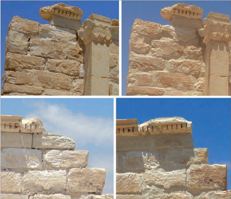
Fig. 8A. Commemorative monument before and after commencement of work in the 2018 season: details of the wall (Polish–Egyptian Conservation Mission | photos W. Grzegorek)
