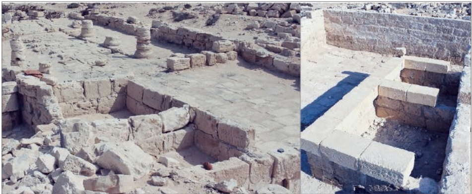
Fig. 2. Plinth of the monument after cleaning (left) and after finishing the walls with a capping at the edge (Polish–Egyptian Conservation Mission | photos S. Medeksza)
