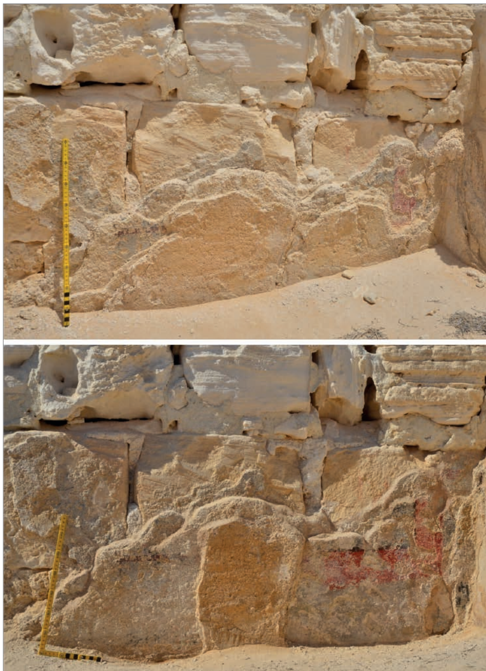
Fig. 3. Northeastern corner of Room 11 in the Roman baths with preserved relics of plaster: top, before conservation; bottom, after conservation; note bands reinforcing the plaster edges (Polish–Egyptian Conservation Mission | photos P. Zambrzycki).
