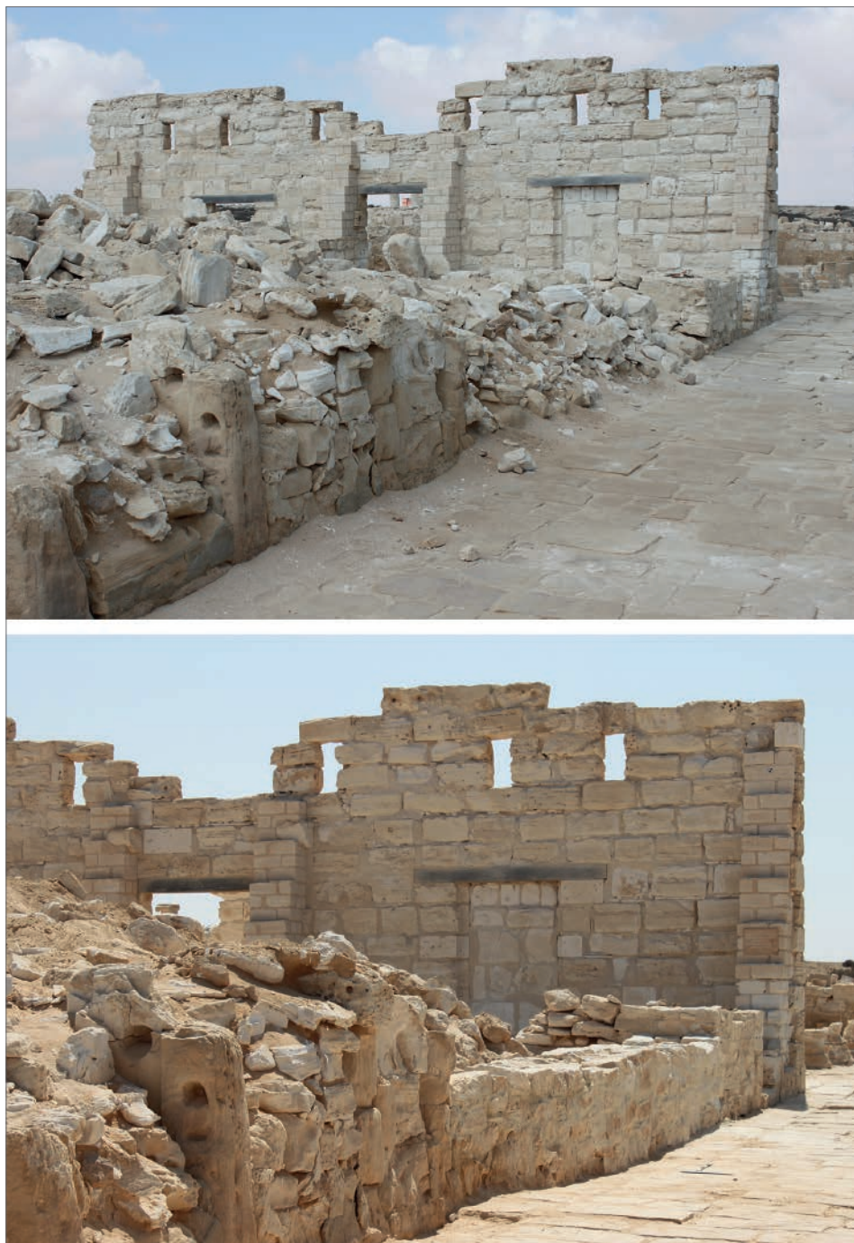
Fig. 5. South side of the street running east from the forum, view from the east: top, before preservation; bottom, after preservation in 2018 (Polish–Egyptian Conservation Mission Marina el-Alamein | photos R. Czerner)
